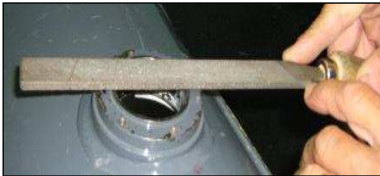
Figure 4: Removing of the paint from the seat ring of the tank
